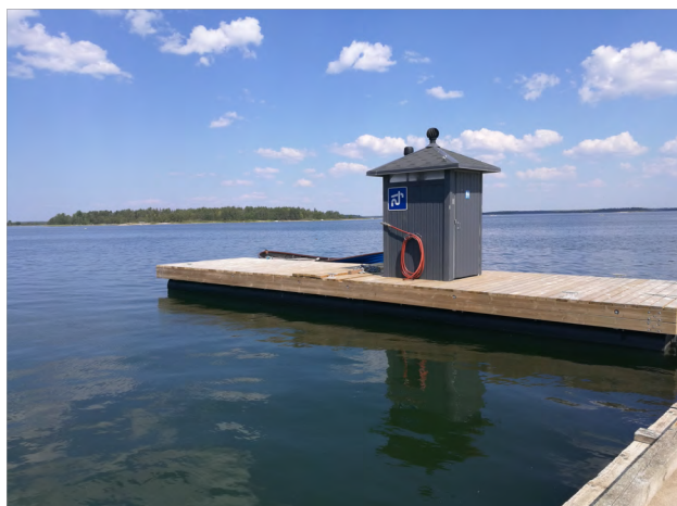
Transportable septic waste water emptying system in Kuuskajaskari island in Rauma.
