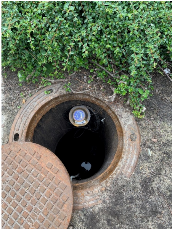
Photo 1. Manhole with channel fill meter.
