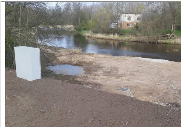
Establishing electric connection for the automatic hydrological stations
