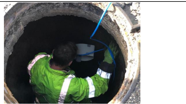
Jurmala_section B_Melluži district_installation of flow meter in waste water manhole
