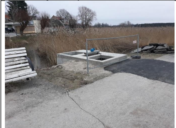
Base for installing smart weirwall
