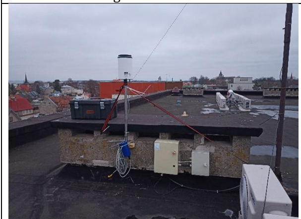
Automatic precipitation monitoring station on the roof of Haapsalu town government
