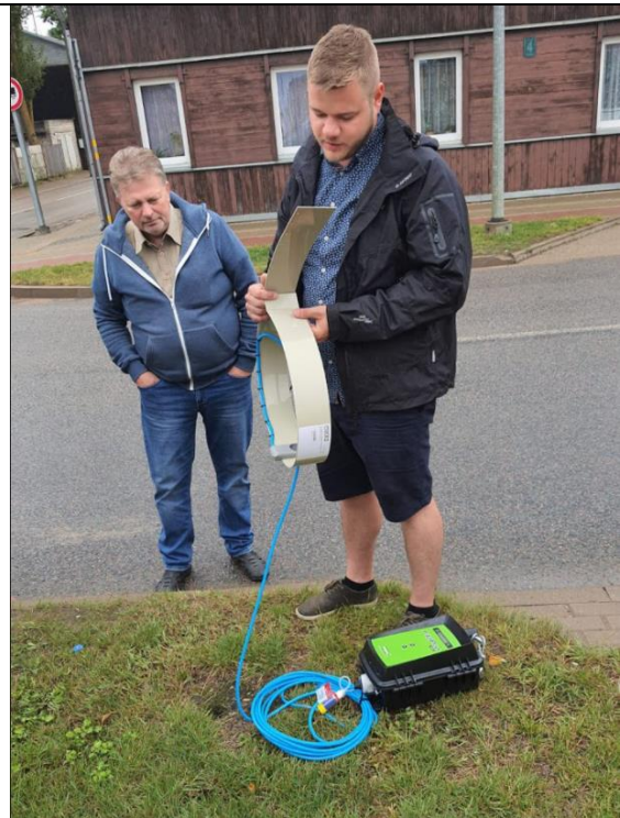
Installing monitoring equipment
