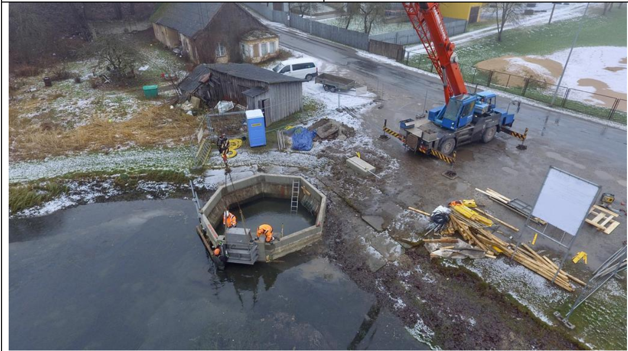
Instalment of the smart weirwall
