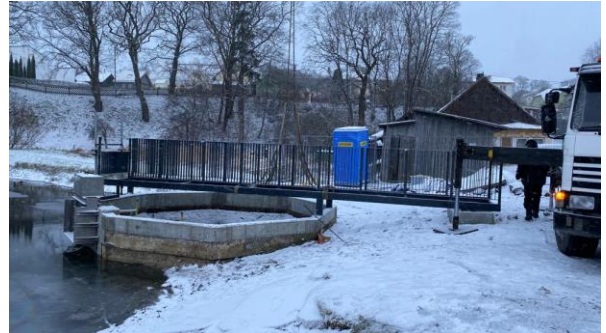
Instalment of new bridge and base for the weirwall
