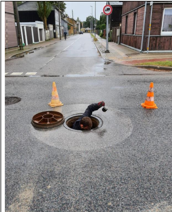
Installing monitoring equipment
