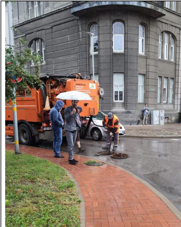
Installing monitoring equipment
