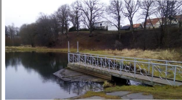
Location of the weirwall prior to the instalment
