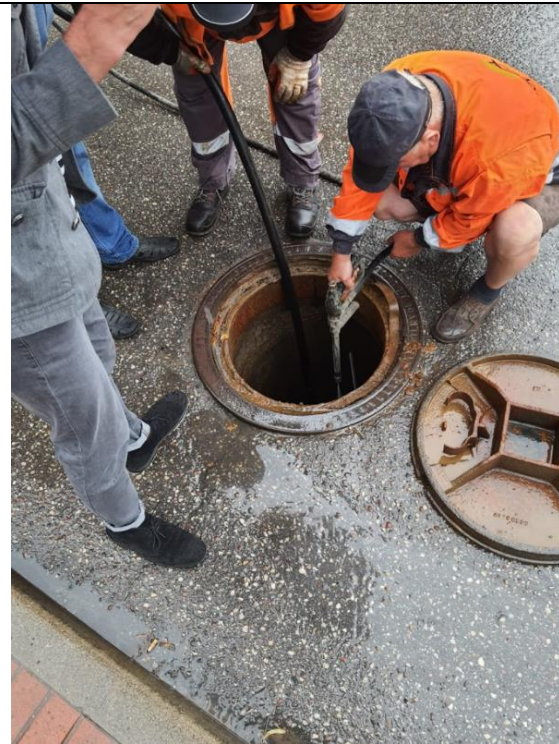
Installing monitoring equipment
